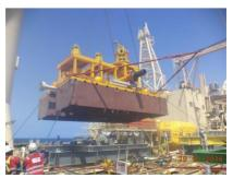
Attendance as MWS onboard Vessel "Volantis" for East Anglia 1 North Subsea Export Cable Jetting and Burial using UT-1 trencher.
